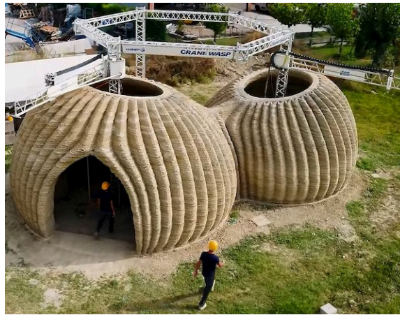
Figure 2.7 AM structures can be created by a deposition head suspended from a gantry system. The system prints the cement or other material layer by layer from the ground up, with the gantry lifting the system as the layers are deposited. (credit: Modification of “The Tecla as of 2021,” by Alfredo Milano/Wikimedia Commons, CC-BY 2.5)
