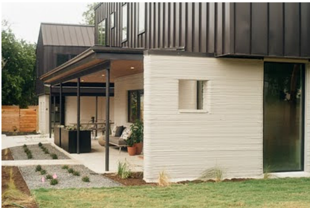
Figure 3.9 3D-printed housing using concrete in the lower floor. (credit: Modification of “3D printed house. Austin, Tx” by Lars Ploughman/Flickr CC BY 2.0).
